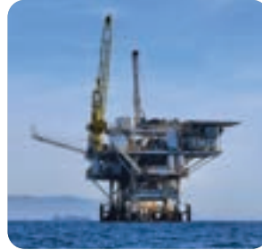
WALKWAYS & HELICOPTER DECKS ON OFFSHORE PLATFORMS
