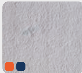
CSP-3 VERY LIGHT SHOT BLASTING OR VERY ROUGH GRINDING
