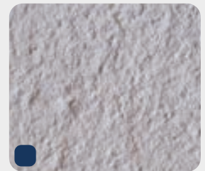
CSP-5 MEDIUM SHOT BLASTING
