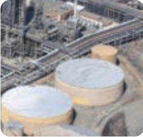
STORAGE TANK BOTTOM PLATES AND ROOF PLATES
