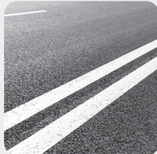
REMOVAL OF MARKINGS
