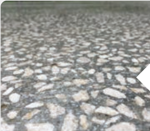
GRINDING WITH BUSH HAMMERED
